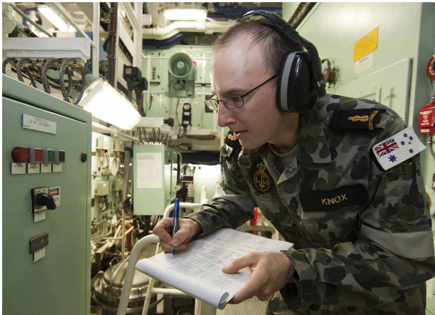
Able Seaman Marine Technician Andrew Knox records the daily readings in the main engine space onboard HMAS Perth.
