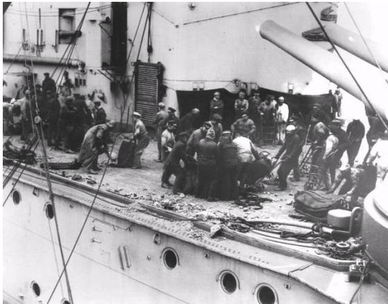
*Coaling the RAN battle cruiser HMAS Australia (I) was an all ship evolution involving most of the ship's company to bring the vital energy source on board. It was a laborious and frequently undertaken task limiting range and endurance.*
